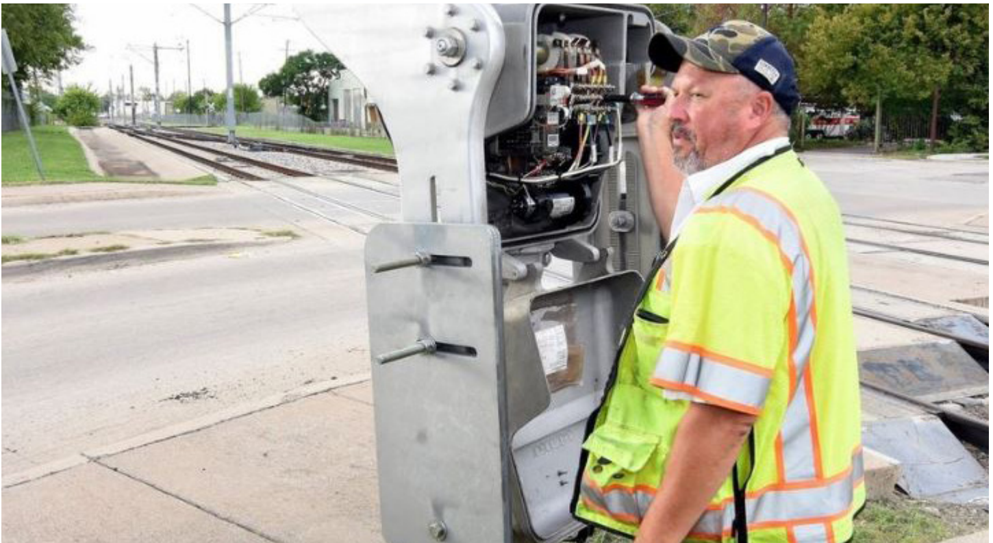
DART Rail At-Grade Crossing
