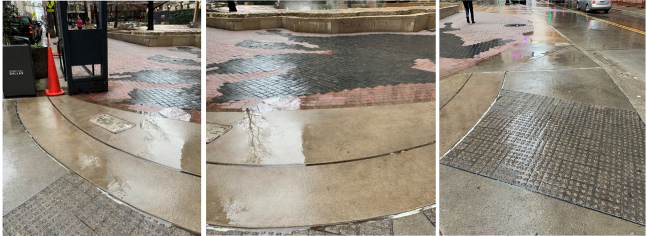
Figure 5.3-B. Curb Ramps at Commerce Street and Lane Street (Proposed Elevator Entrance to Station)
