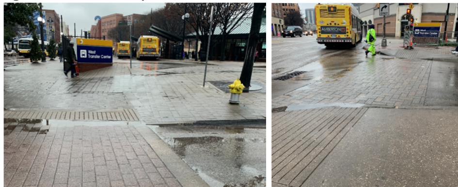
Figure 5.2-B. Curb Ramps at Street Intersections
