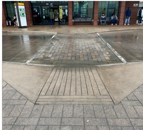
Figure 5.2-A. Curb Ramps at Bus Loading
