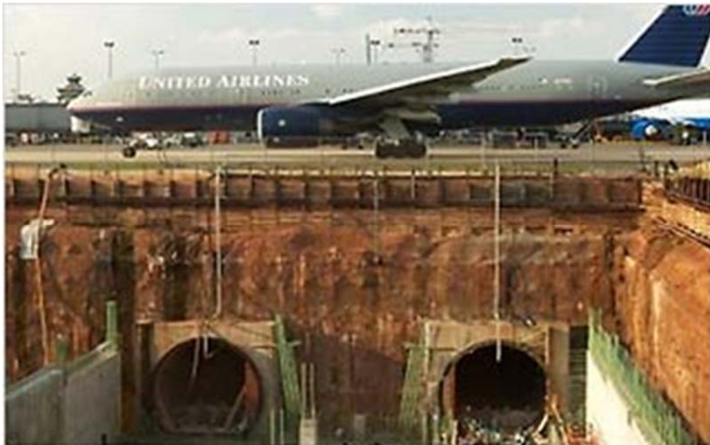
FIGURE 6-4. DULLES AIRPORT TBM TUNNELS
