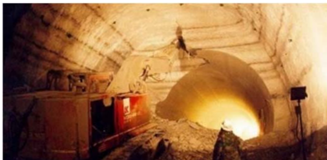
FIGURE 6-2. CITY PLACE STATION ENLARGEMENT VIA ROADHEADER
