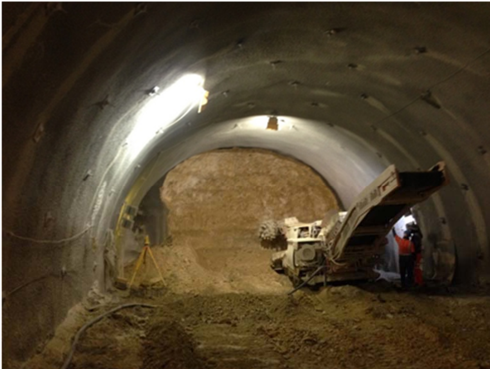
FIGURE 6-8. RIYADH METRO ADIT CONSTRUCTION VIA ROADHEADER
