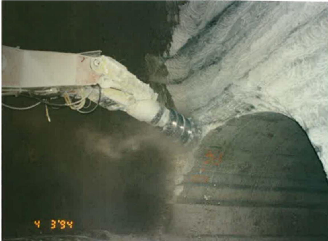
FIGURE 5-12. CITY PLACE STATION CONSTRUCTION, MARCH 1994. AXIAL CUTTING HEAD
