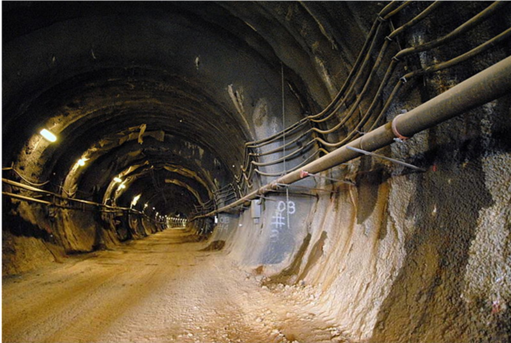
FIGURE 6-3. TYSON'S CORNER SEM TUNNELING – SHOTCRETE INITIAL SUPPORT INSTALLED
