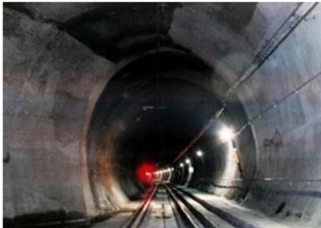
FIGURE 6-2. CITY PLACE STATION ENLARGEMENT VIA ROADHEADER
