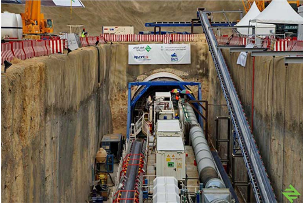
FIGURE 6-7. TBM LAUNCH – RIYADH METRO PROJECT
