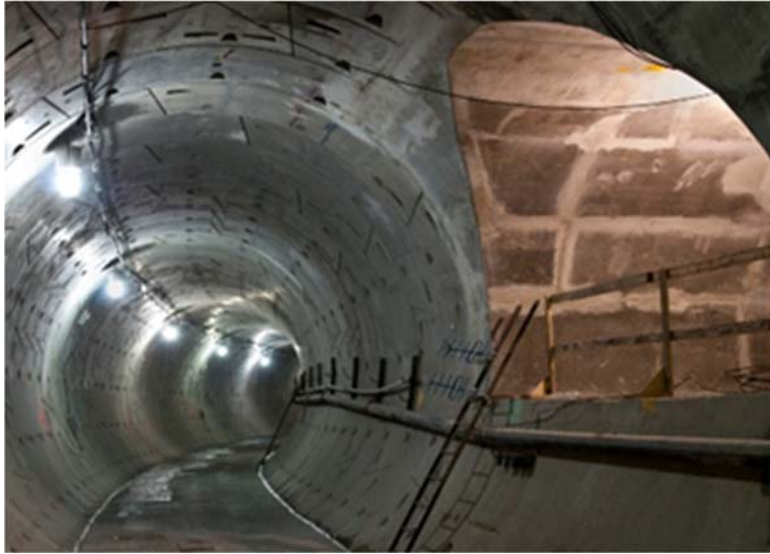
FIGURE 4-7. MTACC'S NUMBER 7 SUBWAY LINE EXTENSION AS-BUILT CROSS PASSAGE
