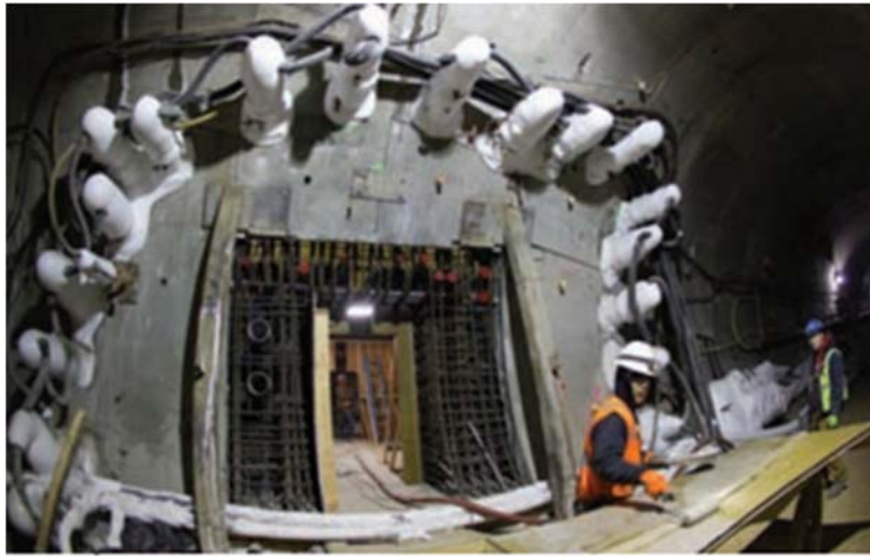
FIGURE 5-4. HORIZONTAL GROUND FREEZING
