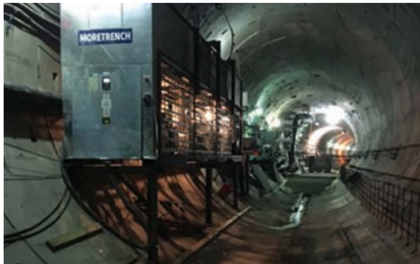
FIGURE 5-5. FREEZE PLANT WITHIN THE TUNNEL
