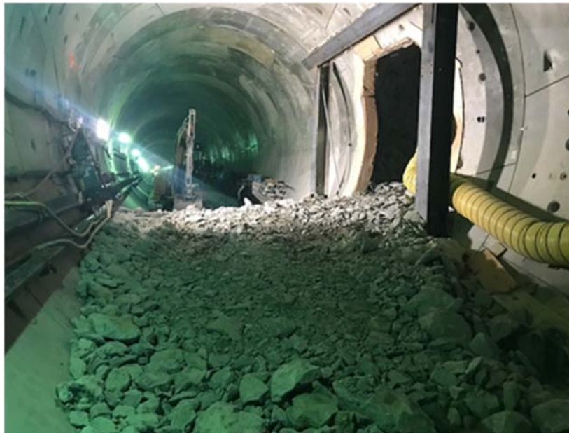
FIGURE 5-1. CRENSHAW CROSS PASSAGE TUNNEL CONSTRUCTION WITHOUT CALIFORNIA SWITCHES
