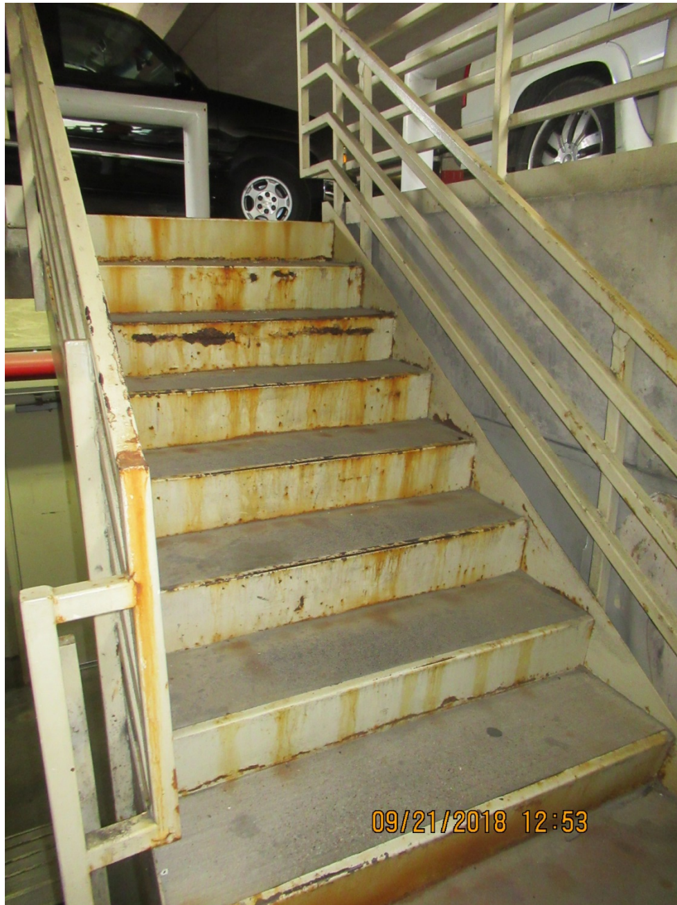
FIGURE 6. VIEW OF TYPICAL DETERIORATION SEEN IN MULTIPLE STAIRWELLS, ACROSS MULTIPLE LEVELS.
