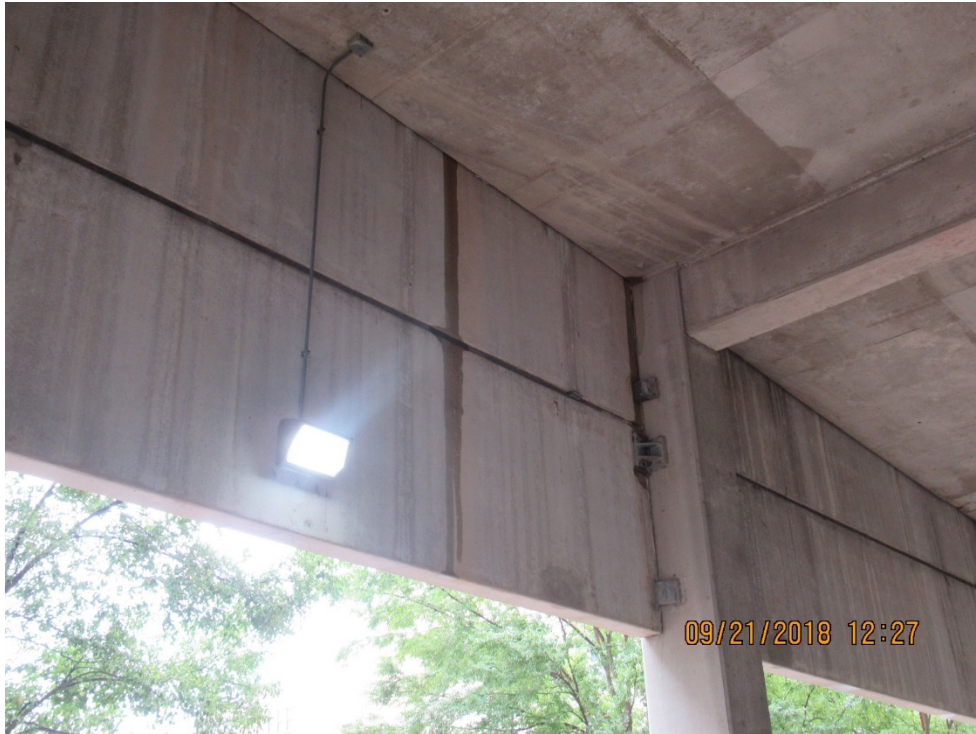
FIGURE A- 6. PRE-CAST CONCRETE CONNECTIONS AT ROOF LEVEL.
