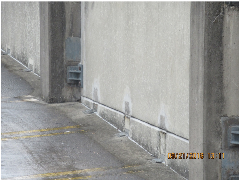
FIGURE A- 6. PRE-CAST CONCRETE CONNECTIONS AT ROOF LEVEL.
