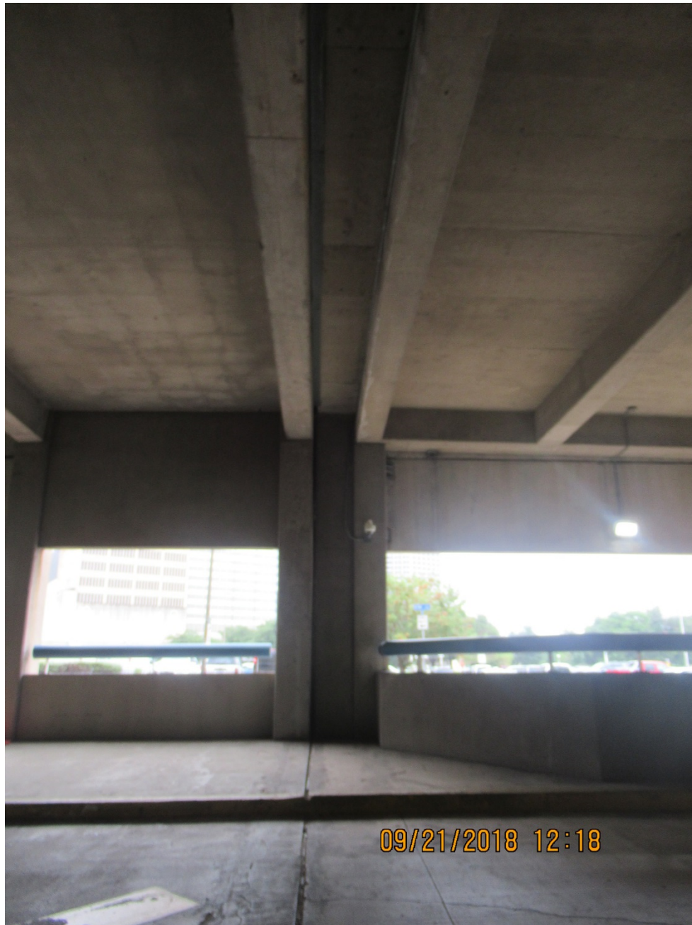
FIGURE A- 2. VIEW OF THE SECTION WHERE THE PARKING GARAGE STRUCTURES MEET.
