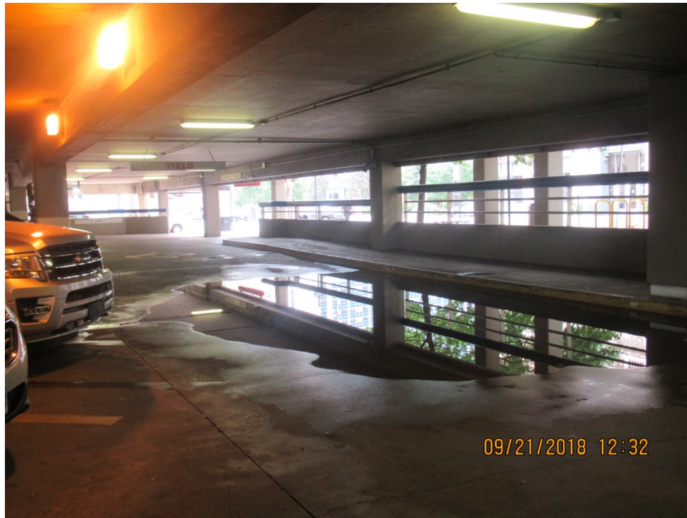
FIGURE 8. VIEW OF PONDING WITHIN THE GARAGE WHERE THERE IS NO DRAIN PRESENT.
