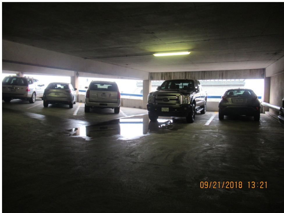
FIGURE 8. VIEW OF PONDING WITHIN THE GARAGE WHERE THERE IS NO DRAIN PRESENT.
