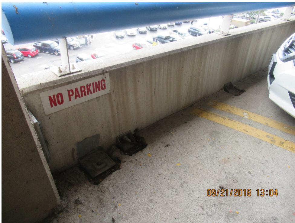
FIGURE 3. VIEW OF TYPICAL CONNECTIONS FOR THE PRE-CAST SLABS.
