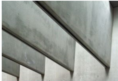
CEILING FINISH 01 ENTRY PAVILION CEILING (MAIN & SECONDARY) Material: Exposed architectural concrete structure Color: White Surface Finish: Smooth BOD: BPD white precast Alternate: Molded GFRC over steel structure
