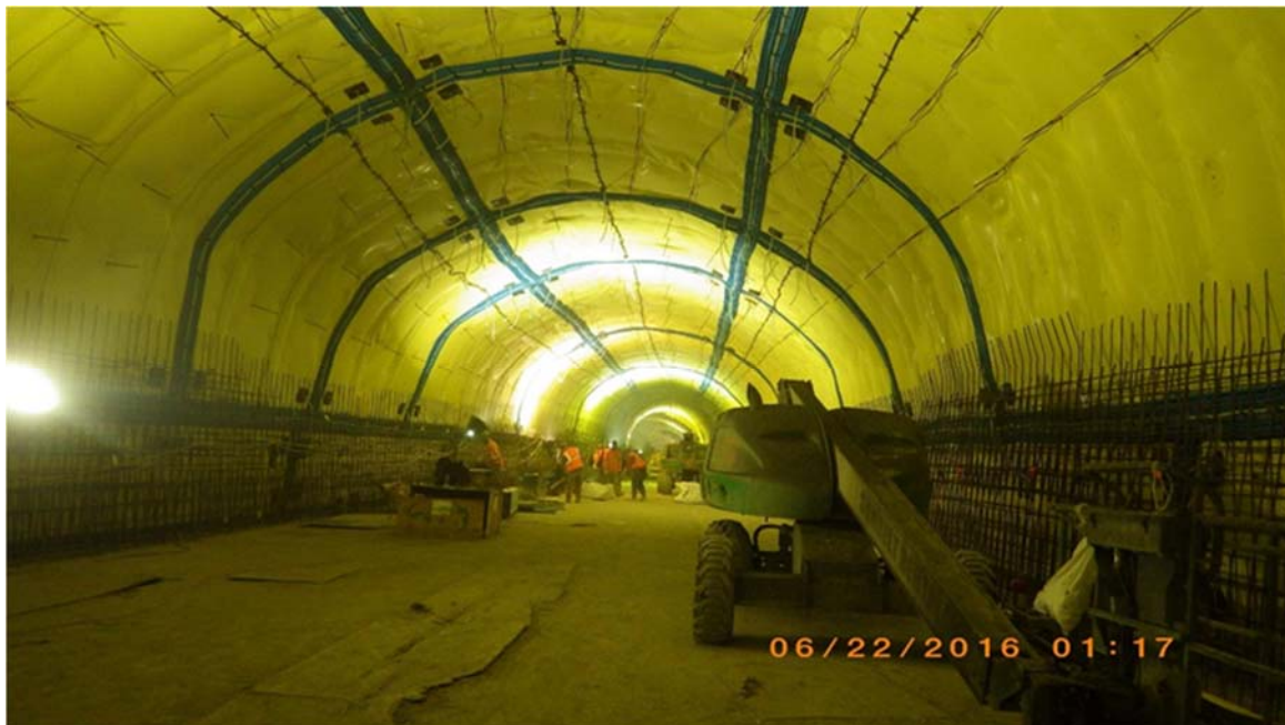
FIGURE 3-8. TYPICAL CONTINUOUS WATERPROOFING (POLYVINYL CHLORIDE - PVC) MEMBRANE COMPARTMENTALIZED SYSTEM (COURTESY OF MTACC FOR EAST SIDE ACCESS PROJECT)
