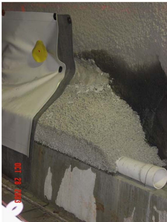
FIGURE 3-2. TYPICAL SIDEWALL DRAINPIPE
