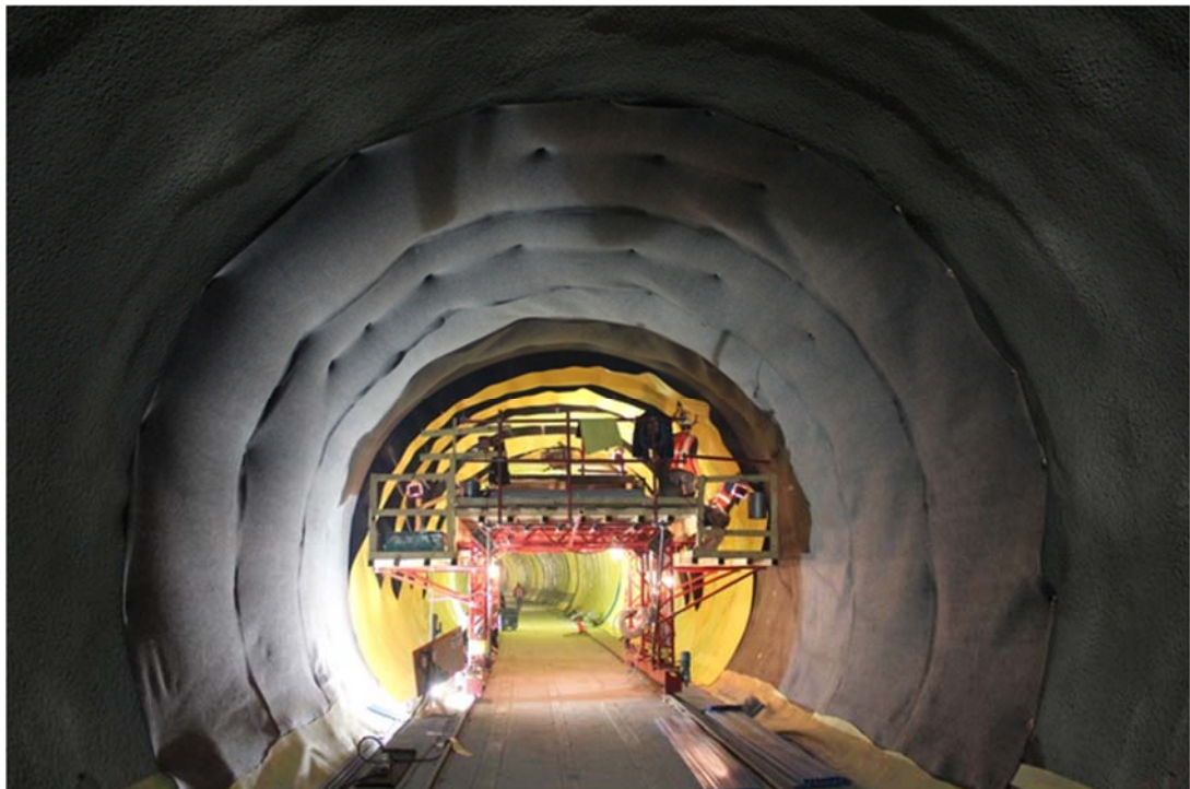
FIGURE 3-10. DRAINAGE LAYER ARCH INSTALLATION
