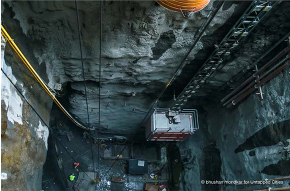
(a) View looking down – shows Alimak, air, water, and discharge lines
