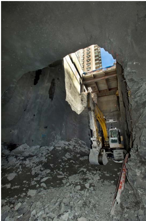
(b) View looking up during excavation of the shaft which is located in Second Avenue. Decking plate above designed to carry automobile traffic.
