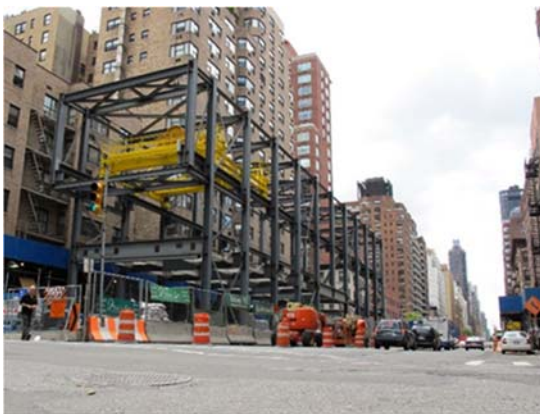
(c) Erection of muck house showing 3 lanes open and 2 lanes closed
