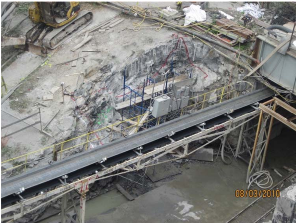
(b) Fixed horizontal belt conveyor at bottom of shaft
