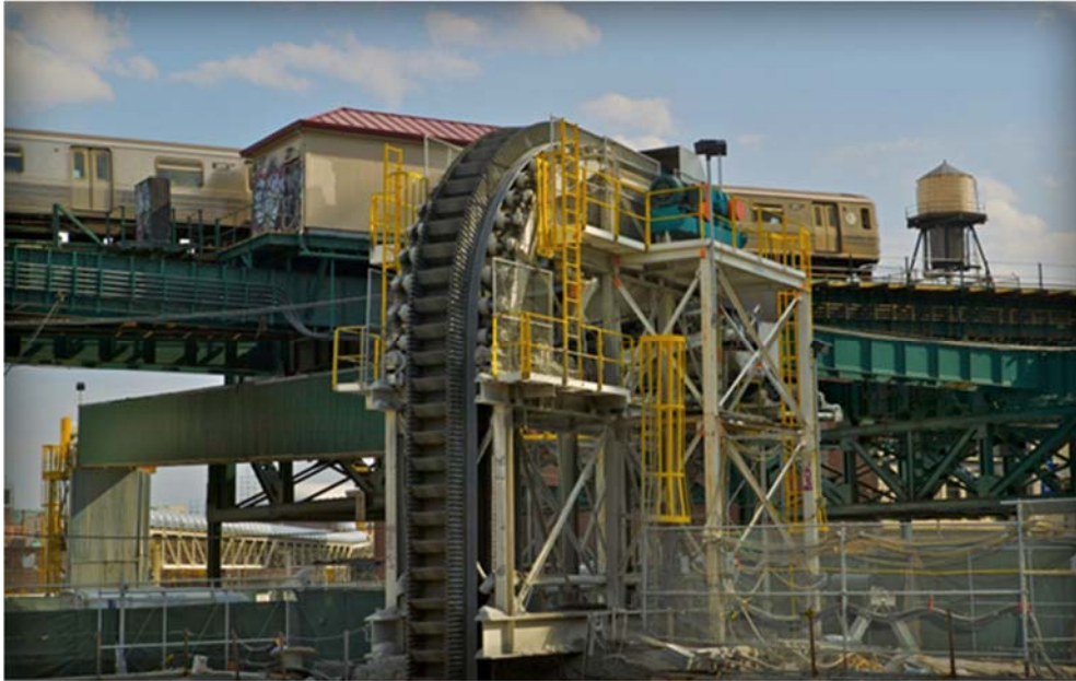
(a) Vertical bucket conveyor at top of shaft
