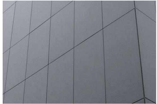
WALL FINISH 04 HORIZONTAL CONNECTOR PASSIVE WALL Material: GFRC cladding Color: Natural concrete color Size: TBD Surface Finish: Smooth BOD Product: FibreC Alternate: Architectural cast-in-place concrete
