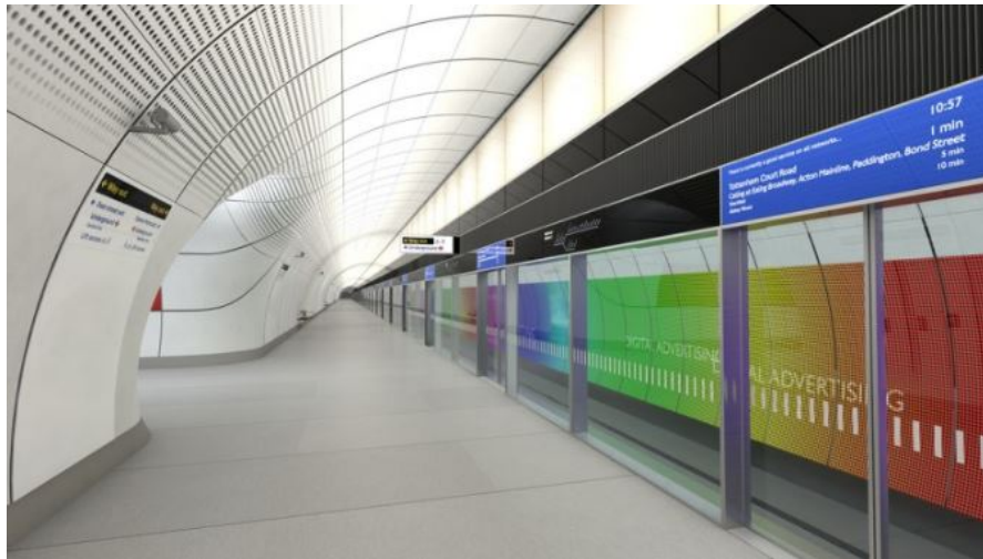
Platform edge doors with integrated signage, utilities and lighting – Crossrail UK
