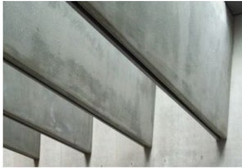
CEILING FINISH 01 ENTRY PAVILION CEILING (MAIN & SECONDARY) Material: Exposed architectural concrete structure Color: White Surface Finish: Smooth BOD: BPD white precast Alternate: Molded GFRC over steel structure
