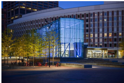
The MBTA Government Center Station is an example of a “glass box” concept that accommodates access from lower levels to the surface with natural light and views to the surrounding urban realm. (Courtesy of HDR)
