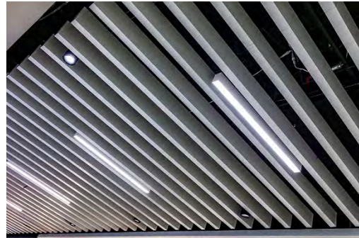
CEILING FINISH 02 HORIZONTAL CONECTOR CEILING Material: Suspended acoustic metal baffle ceiling Color: Grey Surface Finish: Smooth, perforated BOD Product: Linder baffle ceiling, Certainteed Tavola
