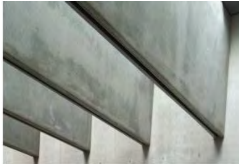
CEILING FINISH 01 ENTRY PAVILION CEILING (MAIN & SECONDARY) Material: Exposed architectural concrete structure Color: White Surface Finish: Smooth BOD: BPDF white precast Alternate: Molded GFRC over steel structure
