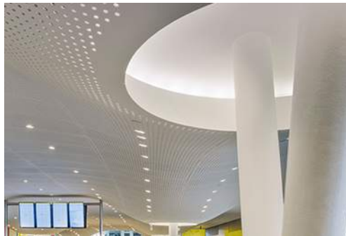
CEILING FINISH 03 PLATFORM SHAFT CEILING Material: Molded GFRC Color: White Surface Finish: Smooth, matte, perforated option BOD Product: Formglas GFRC
