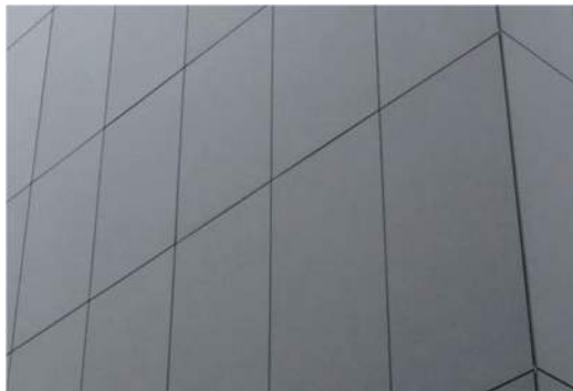
WALL FINISH 01 ENTRY SHAFT TYPICAL WALL Material: GFRC cladding Color: Neutral concrete color Size: TBD Surface Finish: Smooth BOD Product: FibreC
