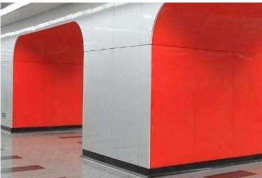
WALL FINISH 06 PLATFORM Material: Vitreous enamel steel Color: Varies at each station Size: TBD Surface Finish: Smooth, glossy BOD Product: PG Bell Alternate: UHPC
