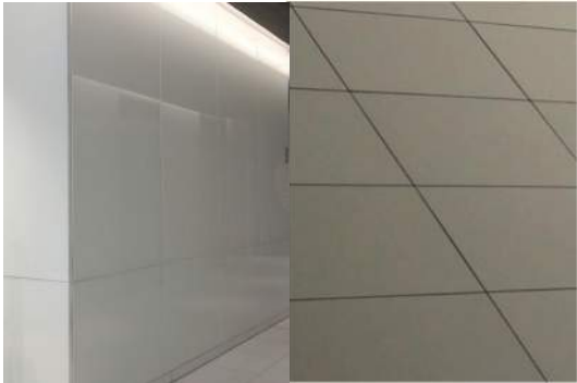
WALL FINISH 05 PLATFORM SHAFT Material: Opaque & clear low iron glass Color: TBD Size: TBD Surface Finish: Smooth, glossy Alternate: Glossy fluted/molded GFRC
