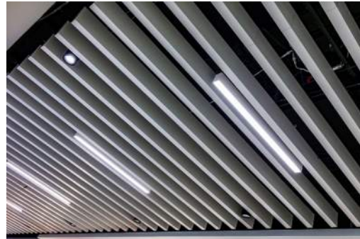
CEILING FINISH 04 PLATFORM CEILING Material: Suspended acoustic metal baffle ceiling Color: Grey Surface Finish: Smooth, perforated BOD Product: Linder baffle ceiling, Certainteed Tavola
