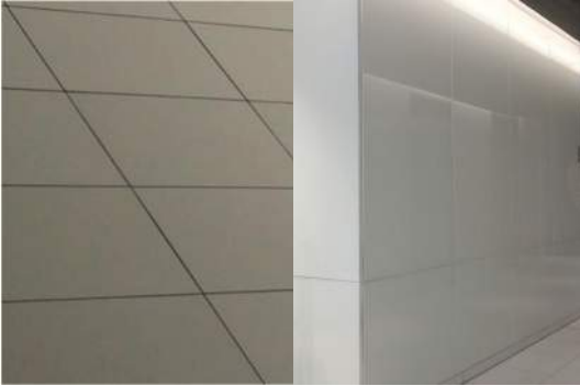
WALL FINISH 03 HORIZONTAL CONNECTOR ACTIVE WALL Material: GFRC cladding Color: Varies at each station Size: TBD Surface Finish: Smooth, glossy BOD Product: FibreC Alternate: Opaque low iron glass
