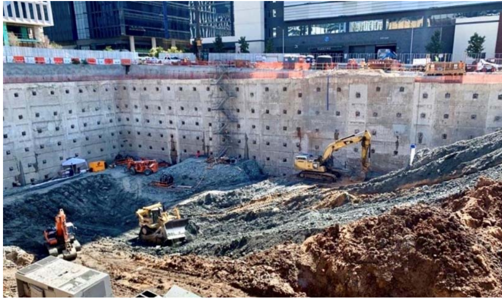
Figure 5-5 Example of Slurry Walls with Anchors for 55-foot deep SOE in Austin, TX (courtesy of Malcom Drilling)
