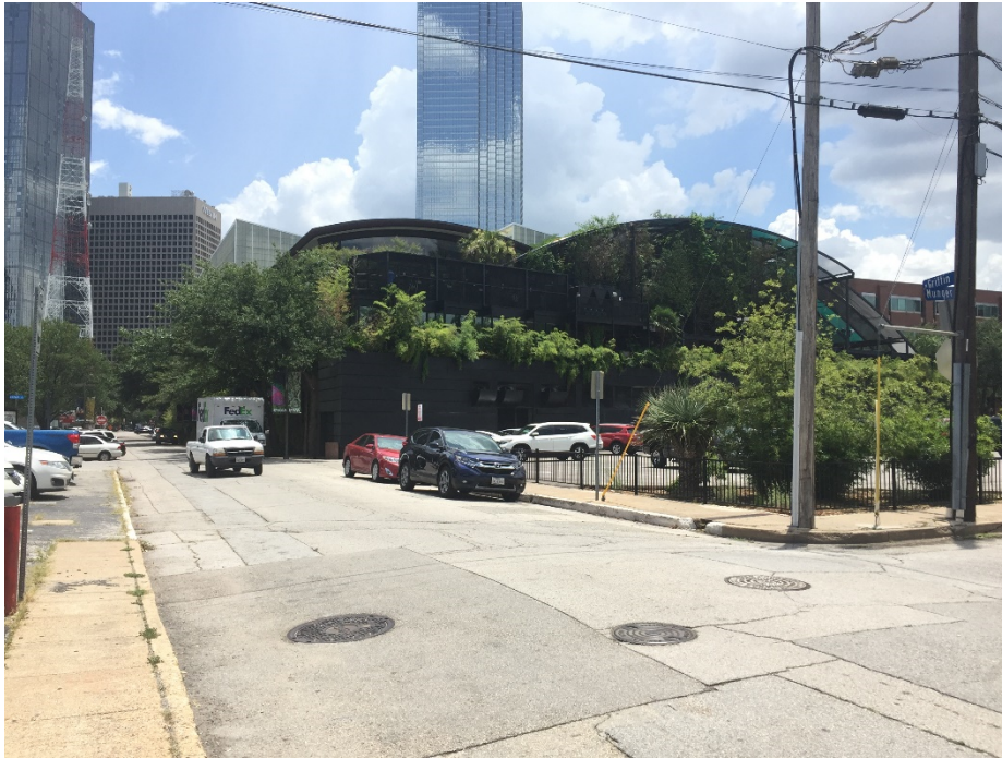
Photo 3. Former location of Graphics Engraving (Map IDs 208 and 212) is located to the right in this photo. View is to the southeast, from N. Griffin St. and Munger Ave.
