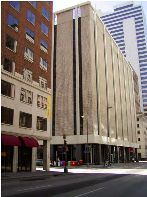
Neiman Marcus Parking Garage (Dal-Park Garage) 1600 block of Commerce Street
