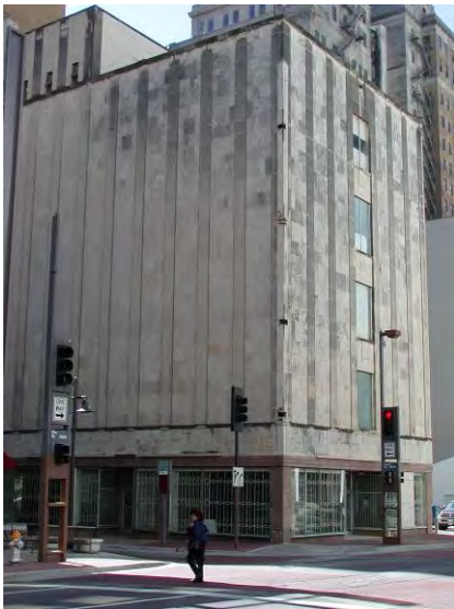
Original building, c. 1955 – 2005
