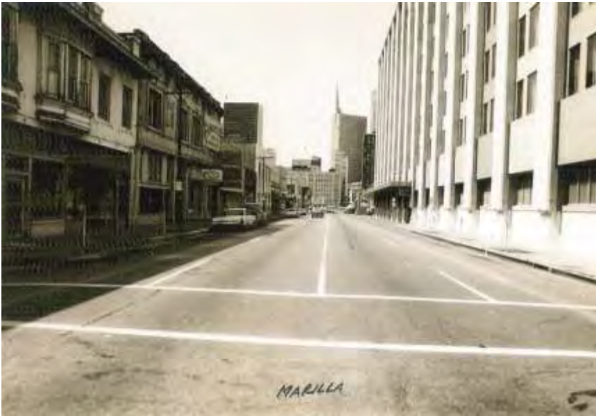
Photograph 7H: South Ervay Street from intersection at Marilla Street. Butler Building is at right; buildings at left side of street have been demolished (site of Dallas City Hall). Camera facing North.
