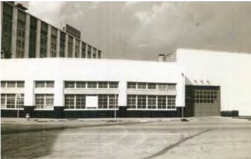
Photograph 6H: Near Marilla Street near intersection at South Ervay; Butler Building is tall building at left; building in foreground has been demolished. Camera facing Northeast.
