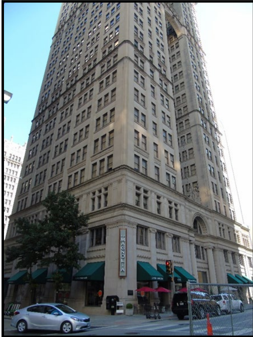
Photograph 2. Magnolia Petroleum Building, 1401 Commerce (aka 108 S Akard) (Resource 15)
