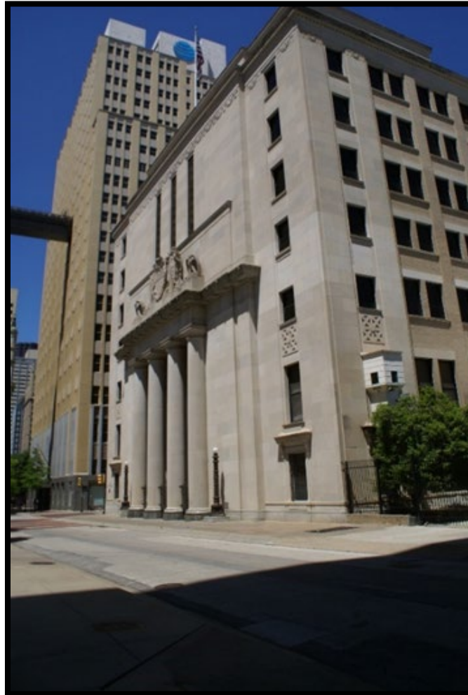
Photograph 5. Federal Reserve Bank, 400 S. Akard (Resource 18)
