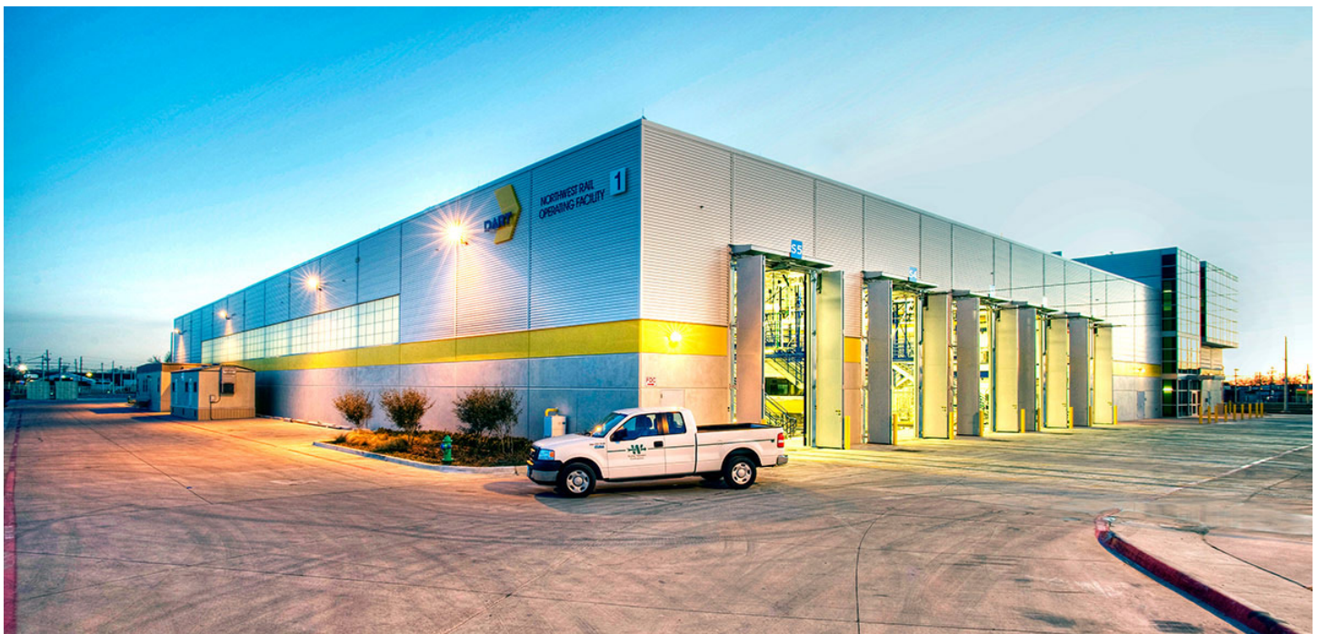
DART Northwest Rail Operations Facility
