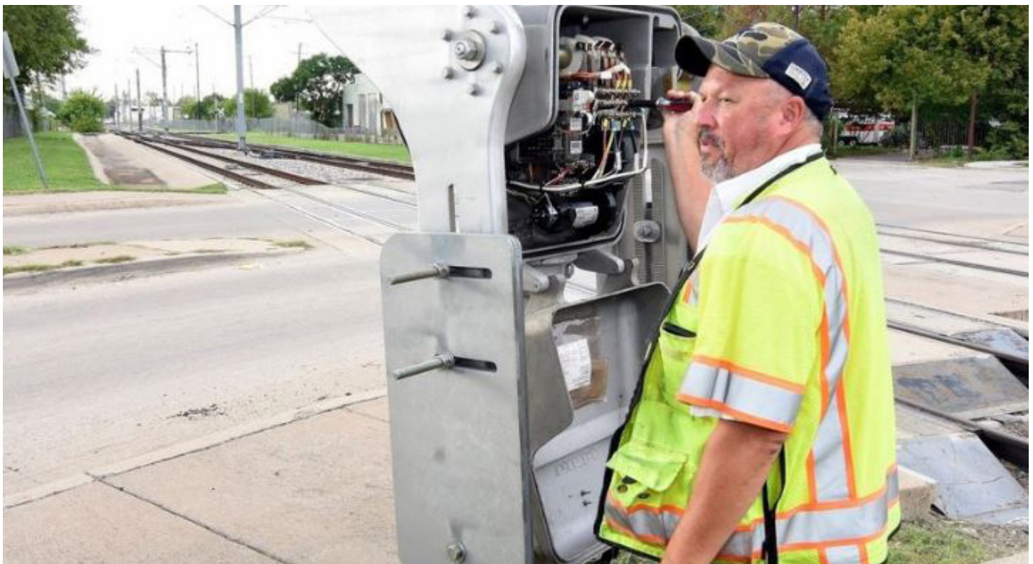
DART Rail At-Grade Crossing
