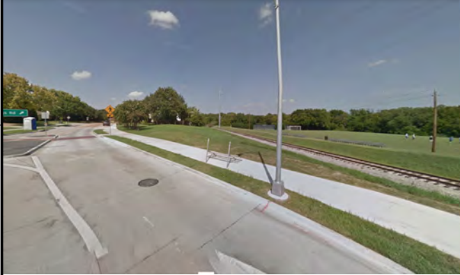
Unit 3A- Area near Preston Road Station
