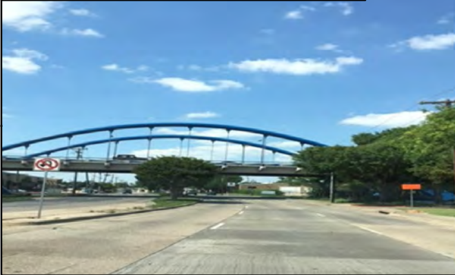
Unit 2B- Wheeler Bridge Over Midway Road
