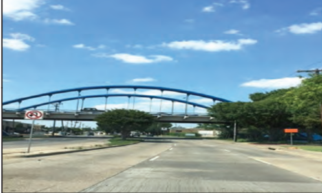
Unit 2B- Wheeler Bridge Over Midway Road
