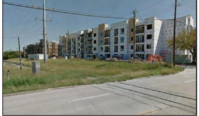
Unit 3A- Multi-Family Complex at Knoll Trail Drive
