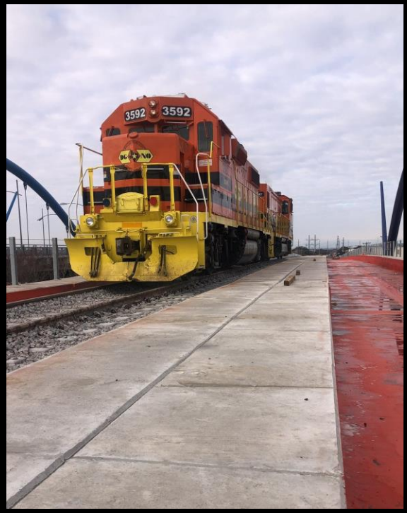
First train run test on Midway Bridge
