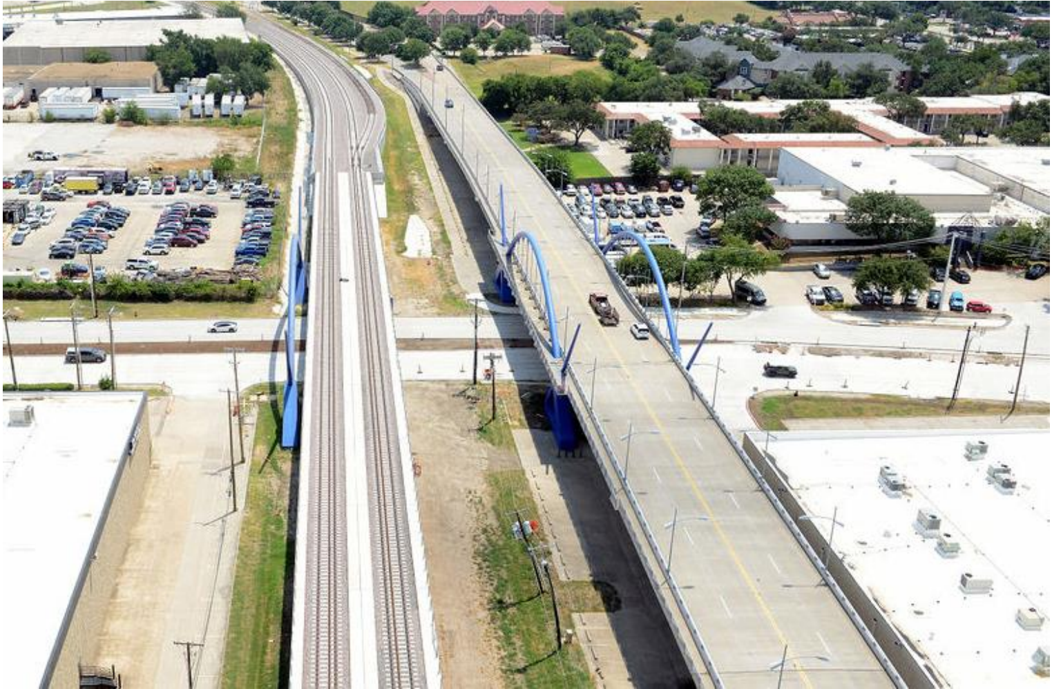
Midway Road Rail Bridge
