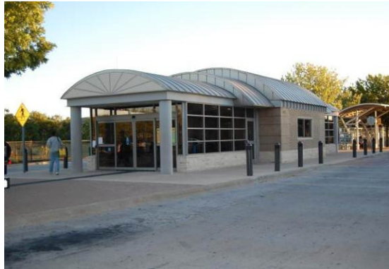
Figure 4-13 Addison Transit Center Waiting Room/Administration Building
